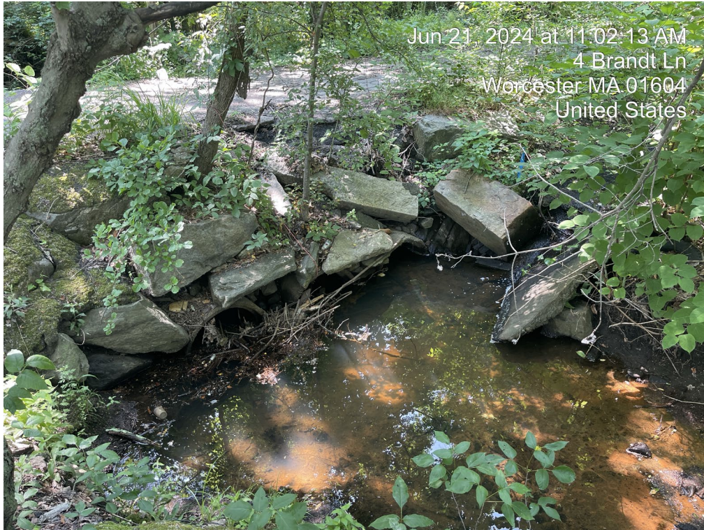
Inlet side of culverts under Brandt Lane (Impact Area 5)
