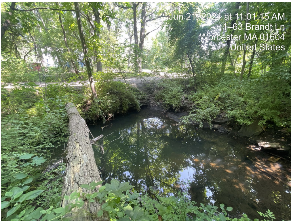
Outlet side of existing culvert under Brandt Lane (Impact Area 6)
