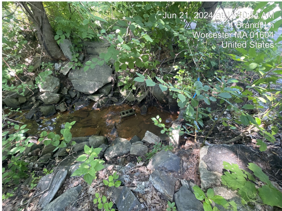
Outlet of culverted stream under site (Impact Area 4)
